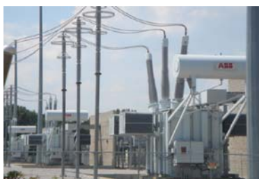
Generator step up transformers (500 kV)
