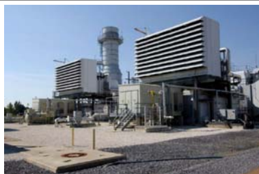
Inlet air filter (self cleaning)
