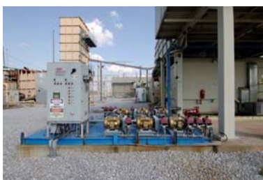
Inlet fogging system
