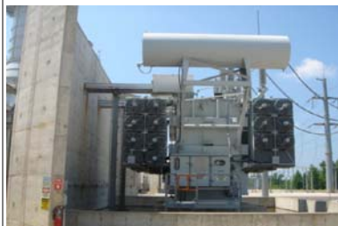
Generator step up transformer (230 kV)
